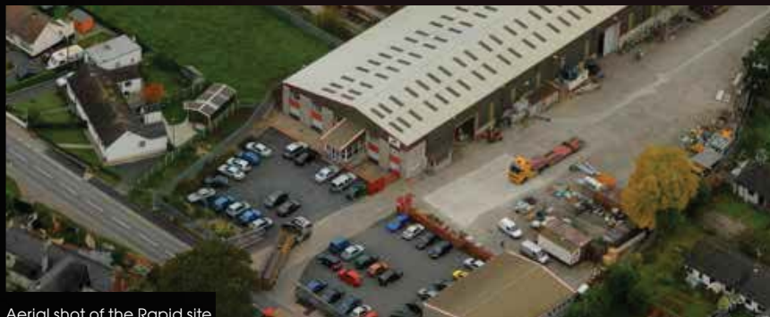
Aerial shot of the Rapid site
